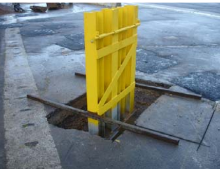
No Deep Footing Required Photograph supplied courtesy of CPNI
