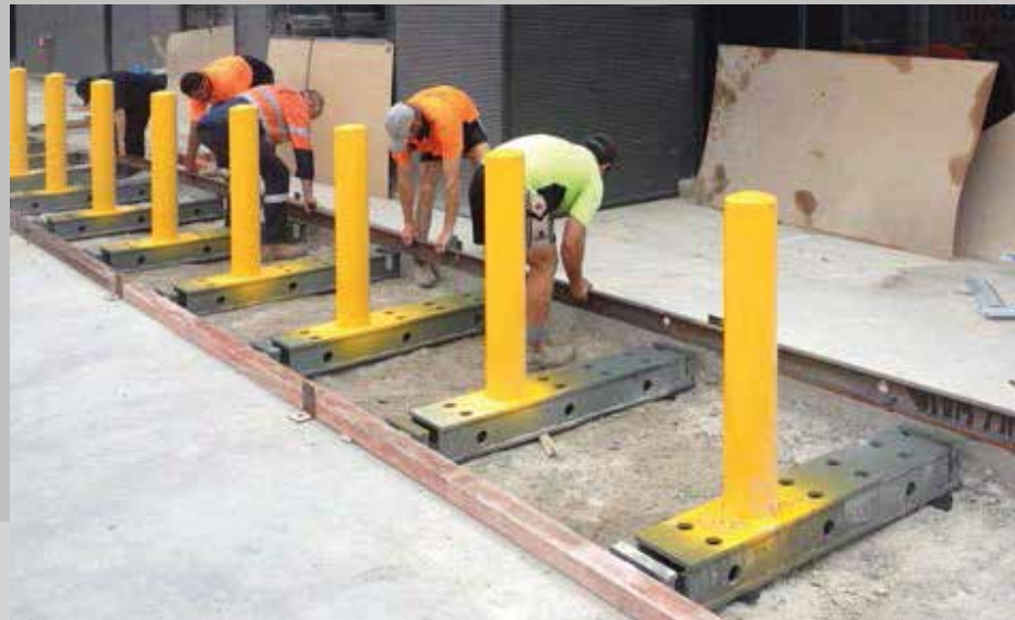
Shallow Mount Concrete Footing Designs for High Security Products
