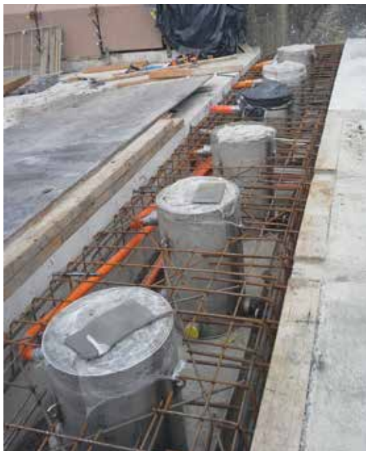
2. Adding Steel Reinforcement
