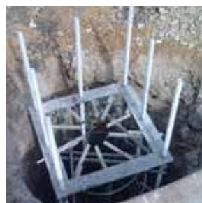
Concrete footings preparation for swing gates
