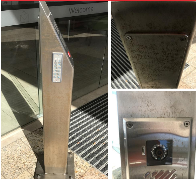
Before - Pics Showing Tea Stain in Bollards
