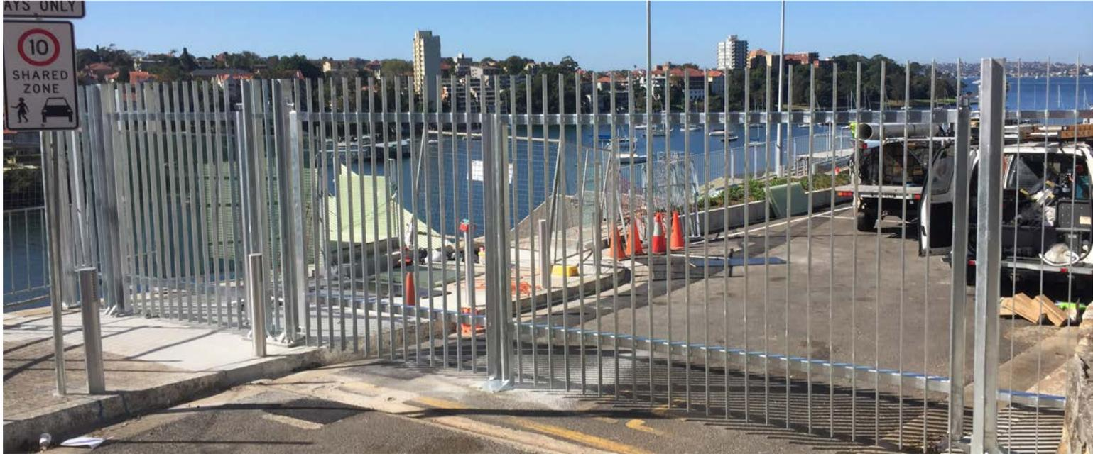
pedestrian bridge will make access to Sydney's ferry network much easier. LEDA have recently manufactured and installed three *pedestrian gates, vehicular swing gates,*
