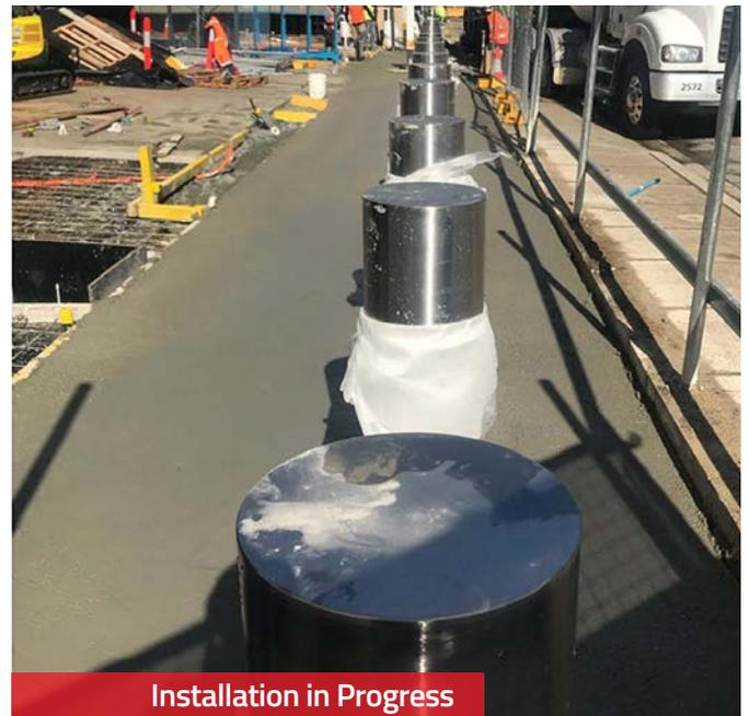
This problem is solved with LEDA's *shallow mount bollard* systems. Requiring only a 114mm deep penetration, LEDA's bollards provide the shallowest footing available in Australia, while still providing a PAS68 rating for a 7.5Tonne vehicle at 80 km/hr.
