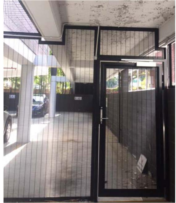
Warrington properties specialises in re-developing medium sized commercial properties. On this project LEDA secured the open underground car park by supplying and installing *security mesh panels* to the perimeter of the building, three track sliding gates for vehicular access and pedestrian access gates.
