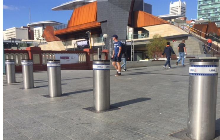
Vehicle access to the site is controlled by two sets of LEDA stainless steel *automatic retractable bollards* which can be controlled and accessed through intercom or card. In this instance our WA office and client chose electro mechanical operated bollards.
