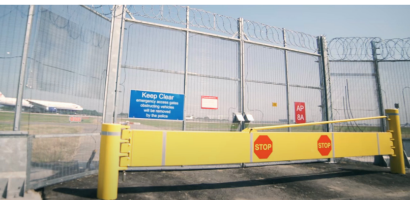
Bollards & Crash Rated Gate Protecting Airport Perimeter
